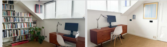
Double glazed window to rear elevation and radiator.
